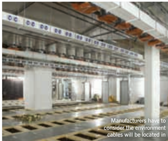
Wire mesh tray is easy to cut and shape on-site using simple hand tools
